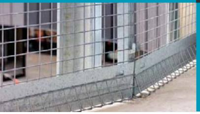
Virtually maintenance free the re-usable galvanised panels and posts are easily installed, removed, transported and stored.
